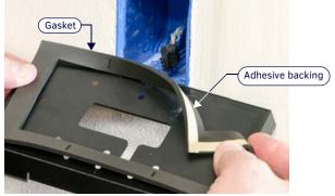
FIG. 4 APPLYING THE OPTIONAL FOAM GASKET TO THE BACK BOX.
